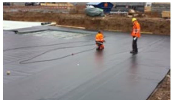
Waterproofing lost formwork installation structure with KÖSTER ECB Membranes
