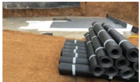
Waterproofing horizontal installation structure with KÖSTER ECB Membranes
