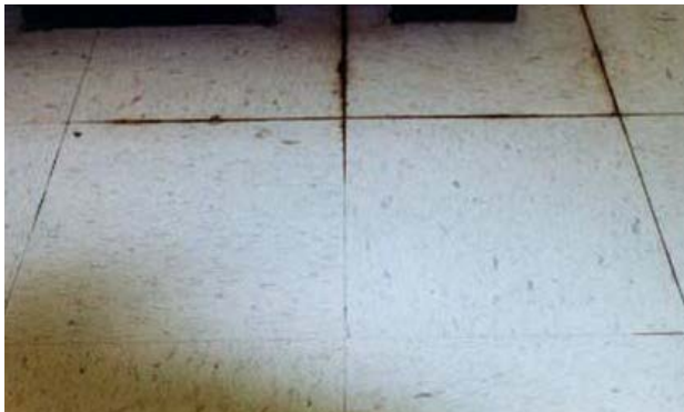
Moisture and high pH values dissolve adhesives ...
