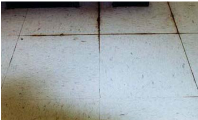
Moisture and high pH values dissolve adhesives ...
