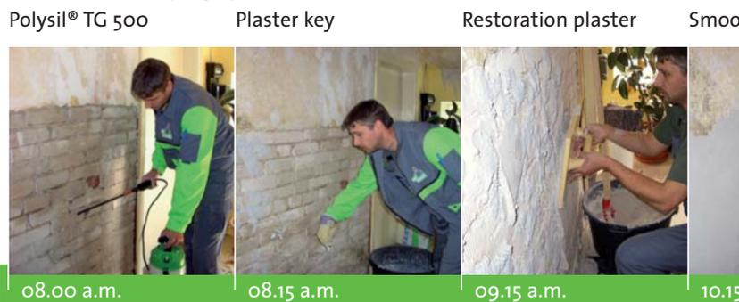
This new fast waterproofing system is the first choice for waterproofing against non-pressurized water and thereby closes the gap between fast waterproofing against pressurized water (negative side waterproofing against leakages with the KD-system) and plain plastering of moist walls with a combination of KÖSTER Polysil® TG 500 and KÖSTER
