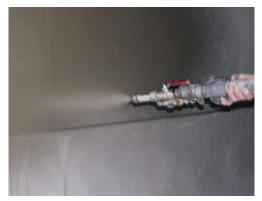
KÖSTER NB 1 Grey can either be applied with a brush or it can be sprayed onto the surface, e.g. with the KÖSTER Peristaltic Pump.
