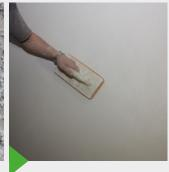
KÖSTER Restoration Plaster is applied to the fully cured key with a trowel or suitable spraying equipment. The surface is then floated smooth.
