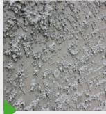
Next, KÖSTER Restoration Plaster Key is applied to ensure optimal adhesion of the KÖSTER Restoration Plaster.
