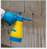
Remove old plaster. Spray KÖSTER Polysil TG 500 onto the surface to block salts and harden the substrate. Fill breakouts and holes with a KÖSTER Repair Mortar.
